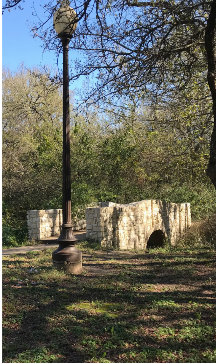
Walkway bridge in Bluebonnet Park
