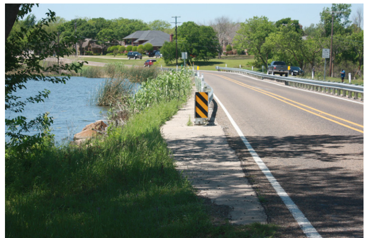
Future improvements call for a pedestrian walkway/trail connection along Country Club Rd across Lake Clark
